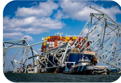
Baltimore Bridge Collapse: U.S. Coal Export Disruptions
