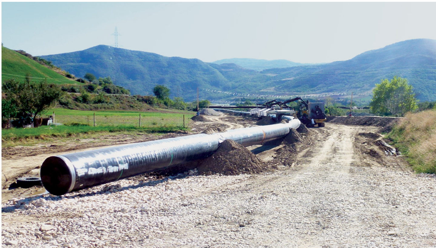
Pipes for the construction of the TAP pipeline through Albania, taken in September 2017. As of September 2018, pipelaying for the onshore portion through Albania is nearly complete. Credit: John Roberts.
